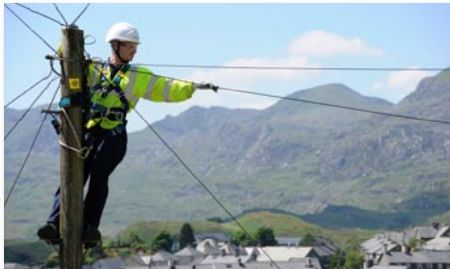
BT Openreach engineer working on Superfast Cymru in Mid Wales.
