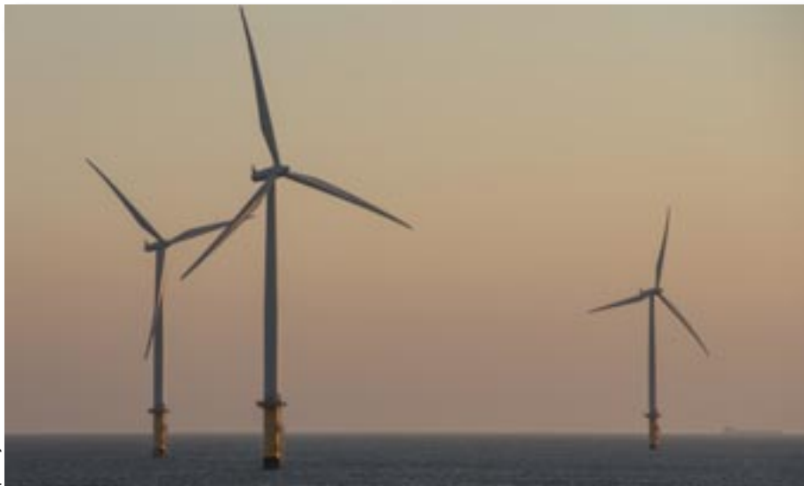
Teesside offshore wind farm, South Gare, Redcar.
