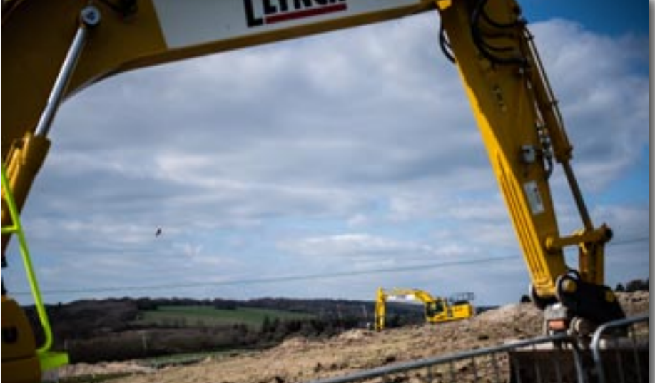
HS2 construction work, Great Missenden, Buckinghamshire.
